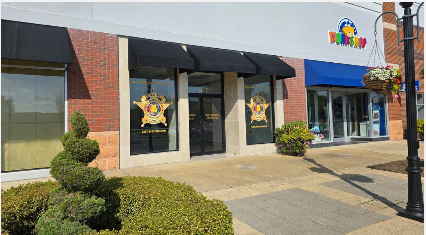
Montgomery County Sheriff's Office Eastchase Substation
