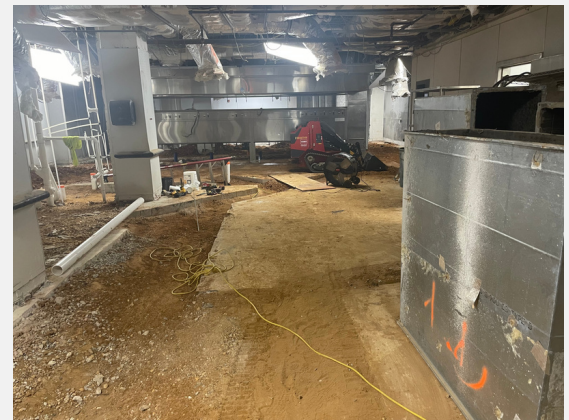
MCDF kitchen renovation.
