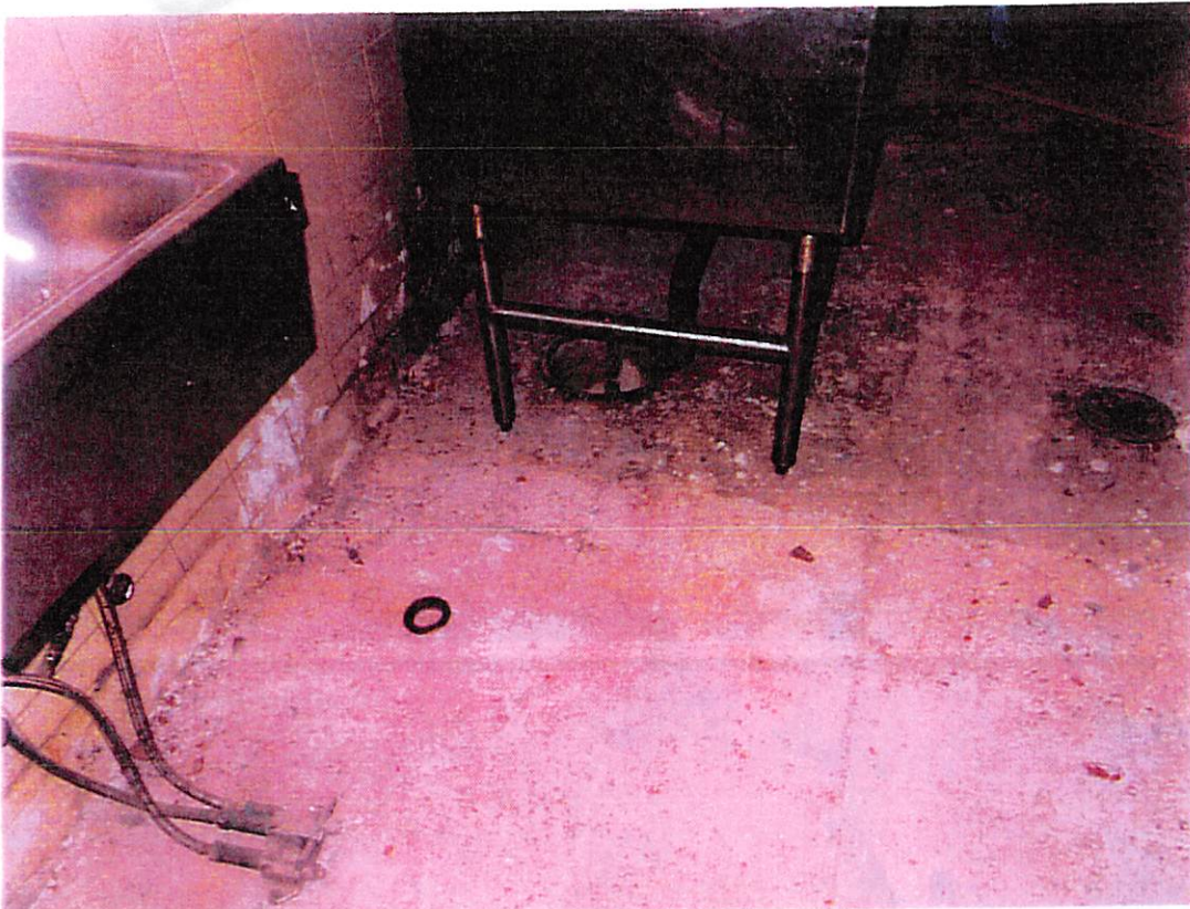
Floor in Kitchen Area
