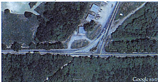
Site 1: Wares Ferry Road at Dozier Road
